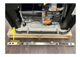
STEP 1: Remove front generator panel and insert lifting rods through generator base lifting holes. Note the rods are shipped with a nut and one washers for each end. Position base rails based on which end you plan to lift from (see label on base).
